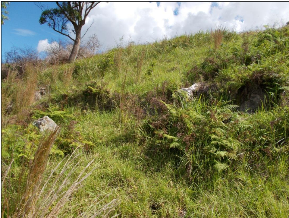
Figure 9: Landslip scarp, north-eastern area
